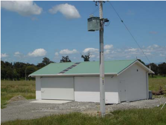
New wastewater building in Featherston
